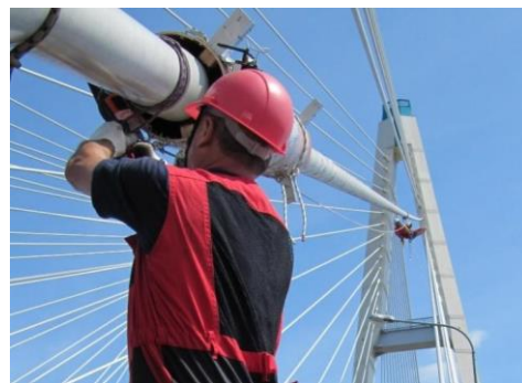
a) Bolshoy Obukhovskiy Bridge across the Neva River
