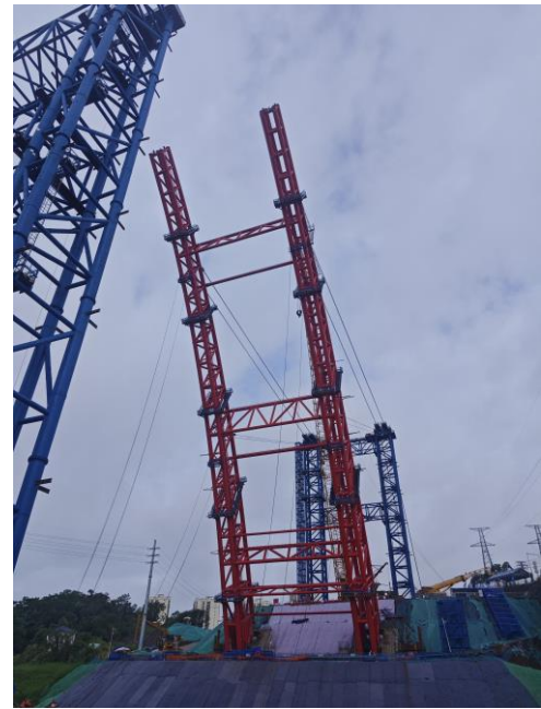
Figure 3 Actual structure at the construction site
