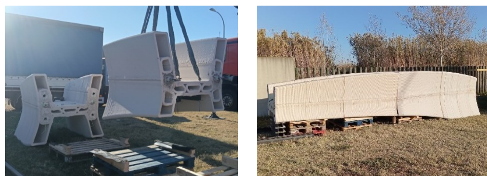
Figure 17 Positioning of the segments and site erection
