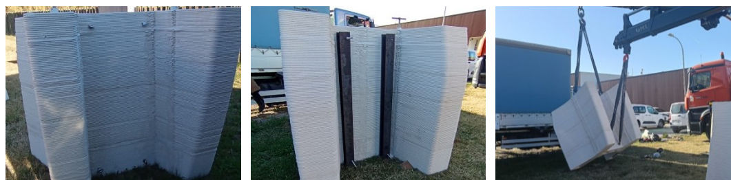
Figure 16 Reorientation procedure
