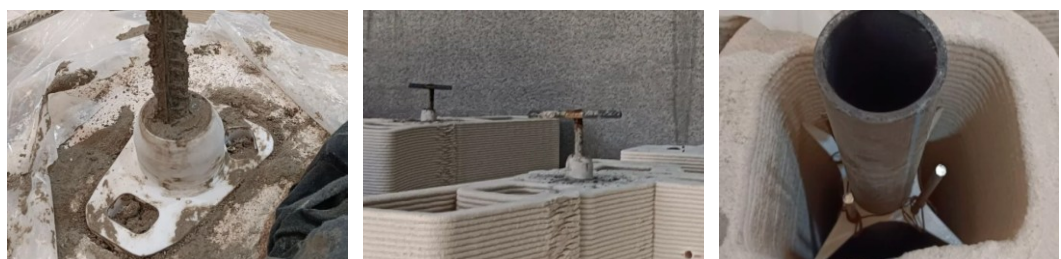
Figure 15 Insertion of T-elements and ducts
