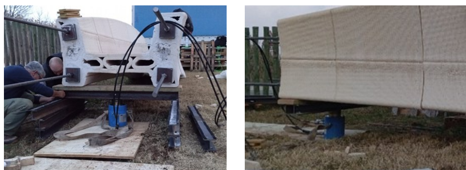
Figure 19 Lifting of the footbridge for support positioning
