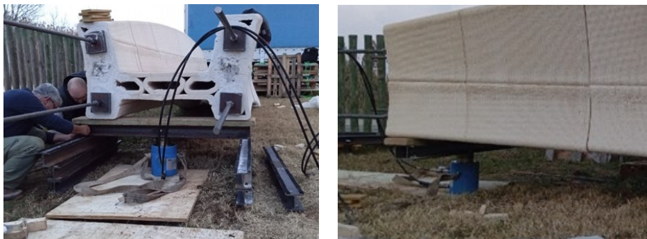
Figure 19 Lifting of the footbridge for support positioning
