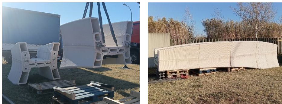
Figure 17 Positioning of the segments and site erection
