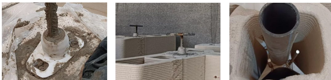
Figure 15 Insertion of T-elements and ducts
