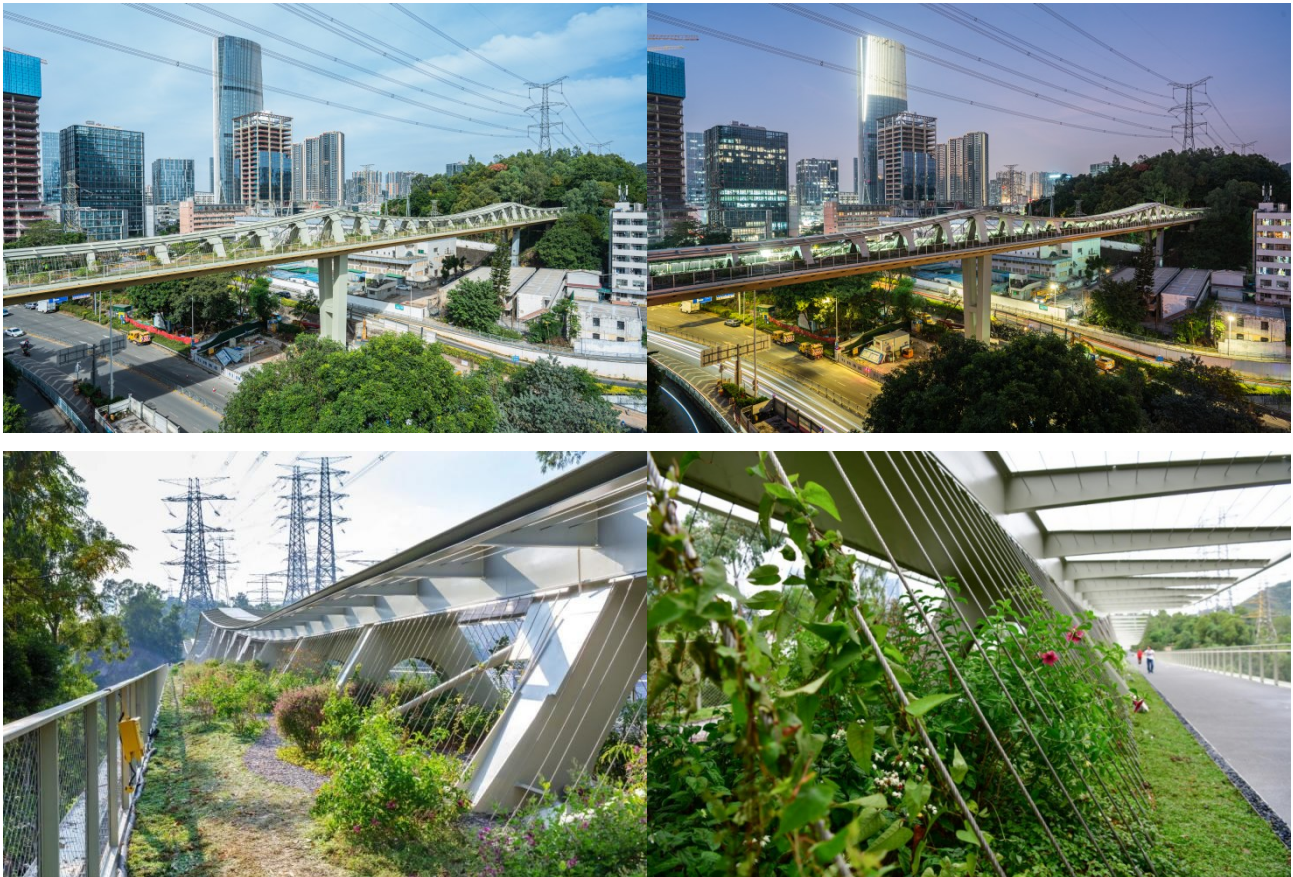
Figure 14 Completed Kunpeng Trail Bridge No. 3
