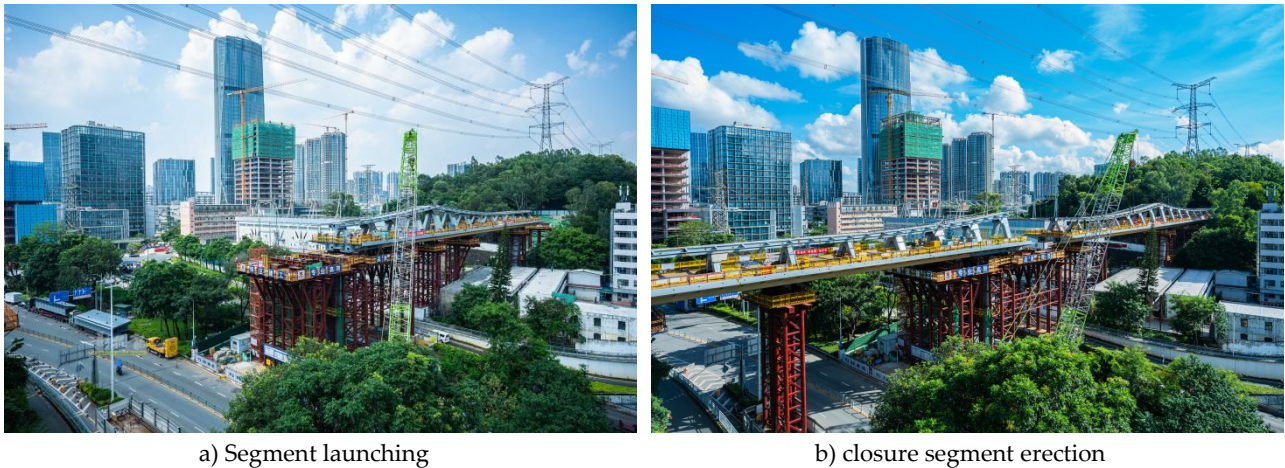
Figure 13 Incremental launching process
