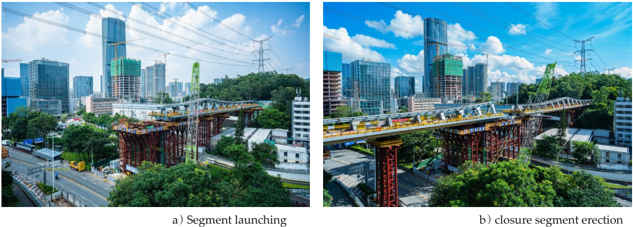
Figure 13 Incremental launching process
