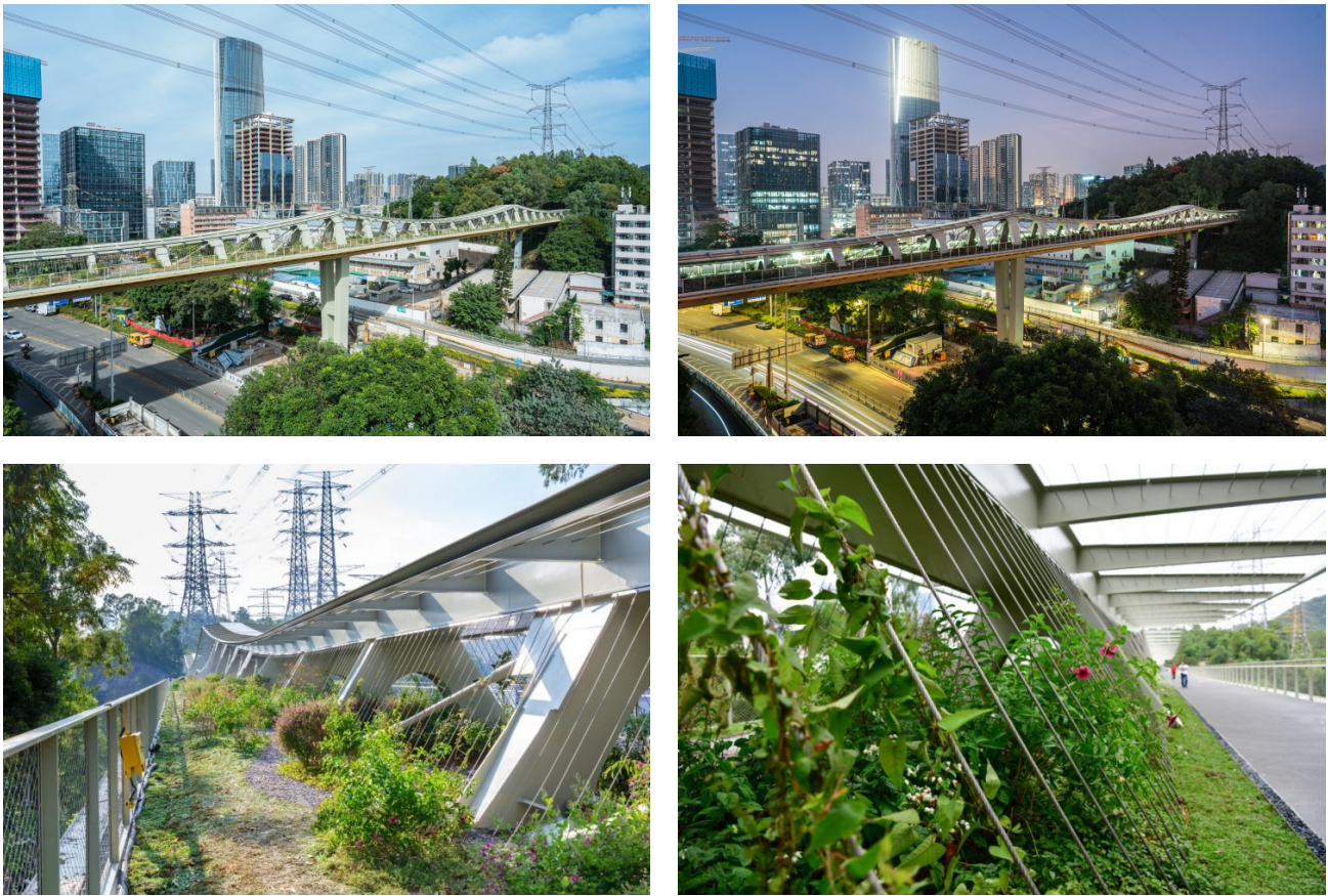
Figure 14 Completed Kunpeng Trail Bridge No. 3
