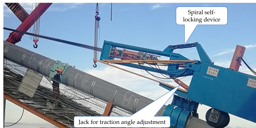
Figure 11 Schematic diagram of the traction angle adjustment device
