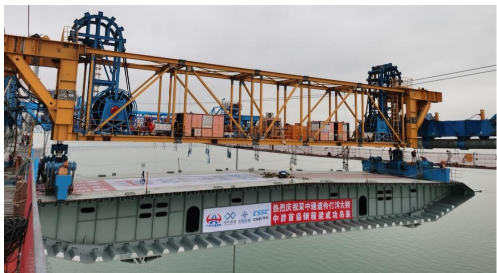
Figure 16 Application of a 1000-ton cable-mounted crane on the Lingdingyang Bridge
