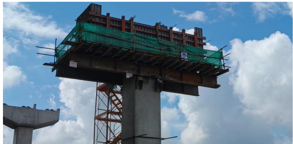
Figure 11 Schematic diagram of the combination of ground-free support and polymer formwork for Jiulong Avenue
