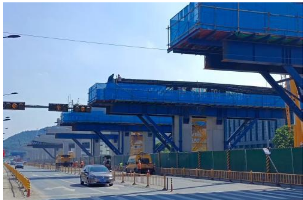
Figure 8 Space beneath the bridge is utilized for social vehicle passage during the construction of the ground-free support system
