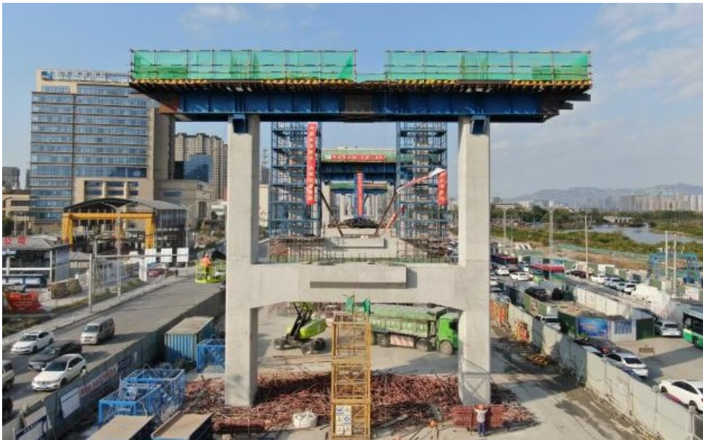
Figure 4 Bent cap formwork support construction for the Wenrui Avenue project
