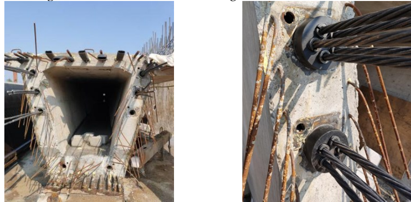
a) End face of a box girder anchorage
