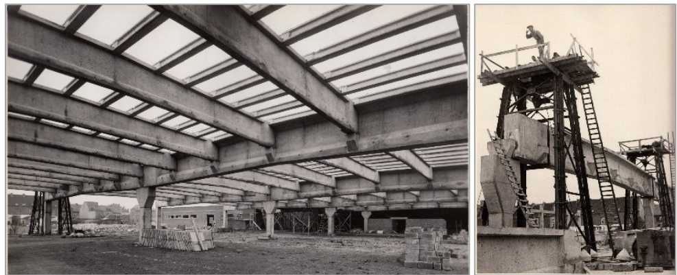
Figure 4 Textile factory with post-tensioned roof beams (1947-1948)
