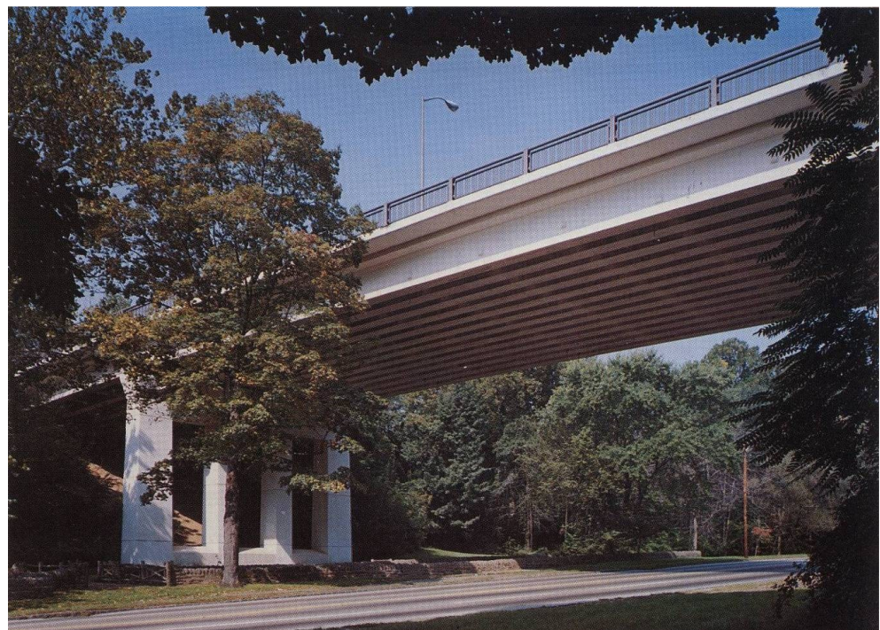
Figure 12 The Walnut Lane Bridge in Philadelphia, USA
