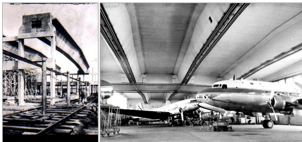
Figure 6 Heavy beams for plane hangar at Melsbroek airport (1949)
