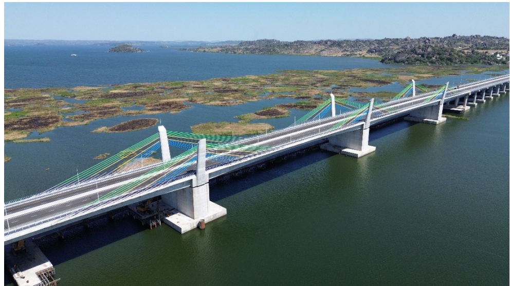
Figure 21 Aerial view showing the overall progress of the project as of April 29, 2025
