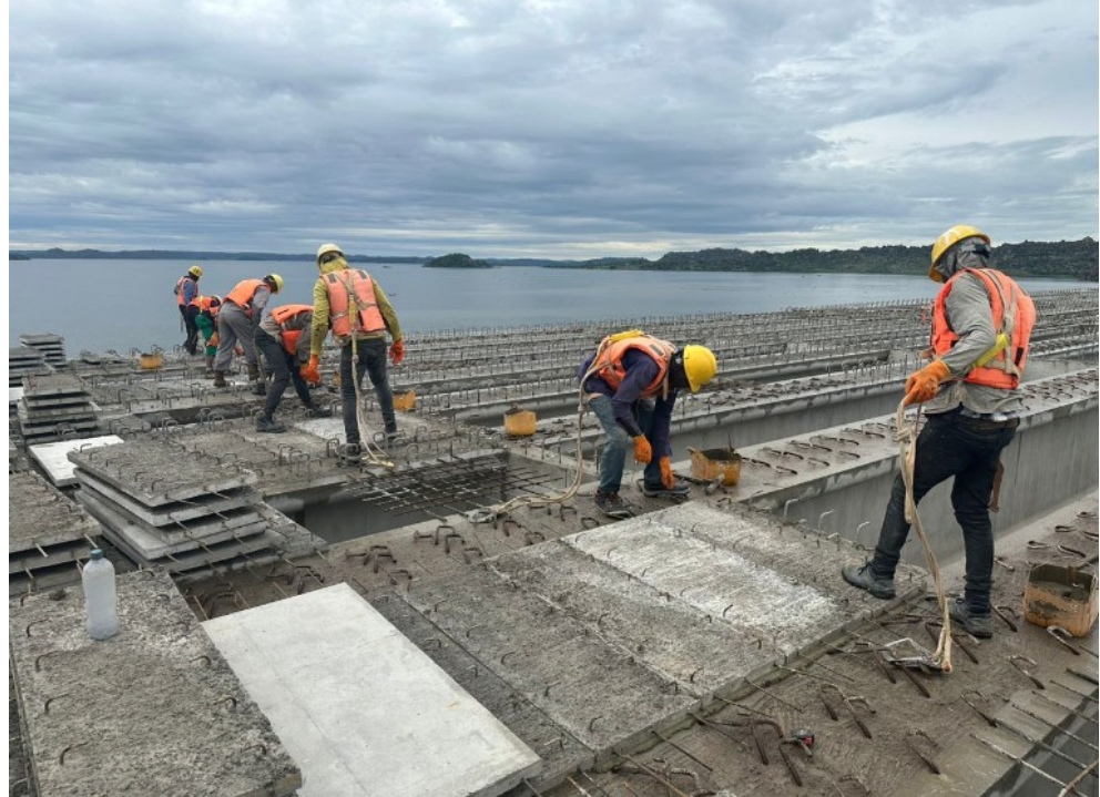
Figure 12 Installation of a precast deck-slab panel and provision of a safe work zone
