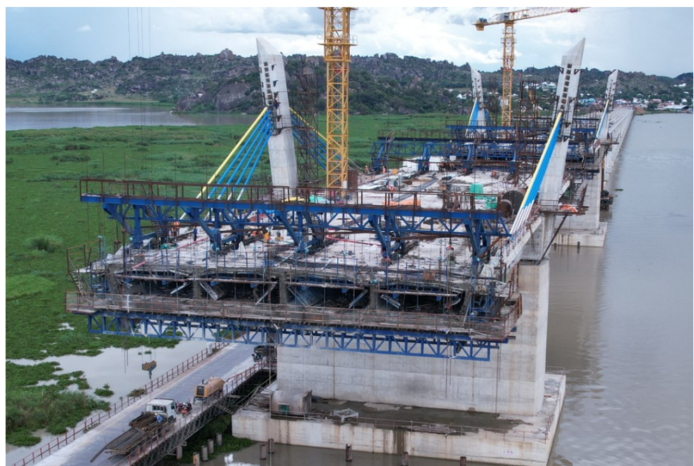
Figure 26 Form-traveller casting standard segments
