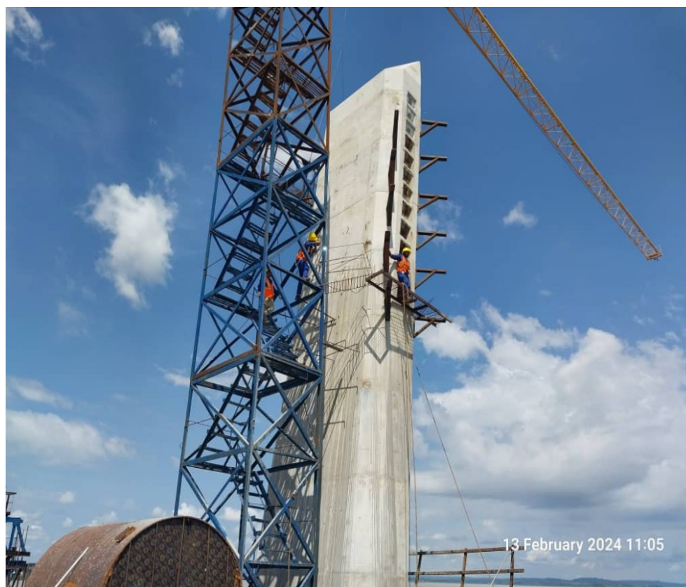
Figure 18 Completed pylon (18.856 m)
