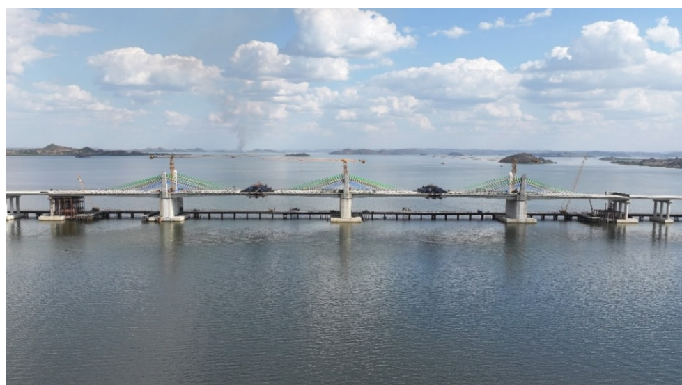
Figure 19 Aerial view showing the overall progress of the project as of 6th October 2024
