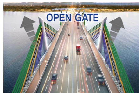
Figure 2 Wide open pylons offering clear vision for drivers
