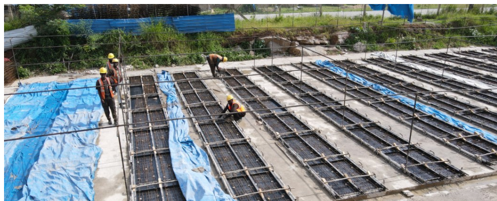
Figure 11 Fabrication yard of the partial slab depth panel
