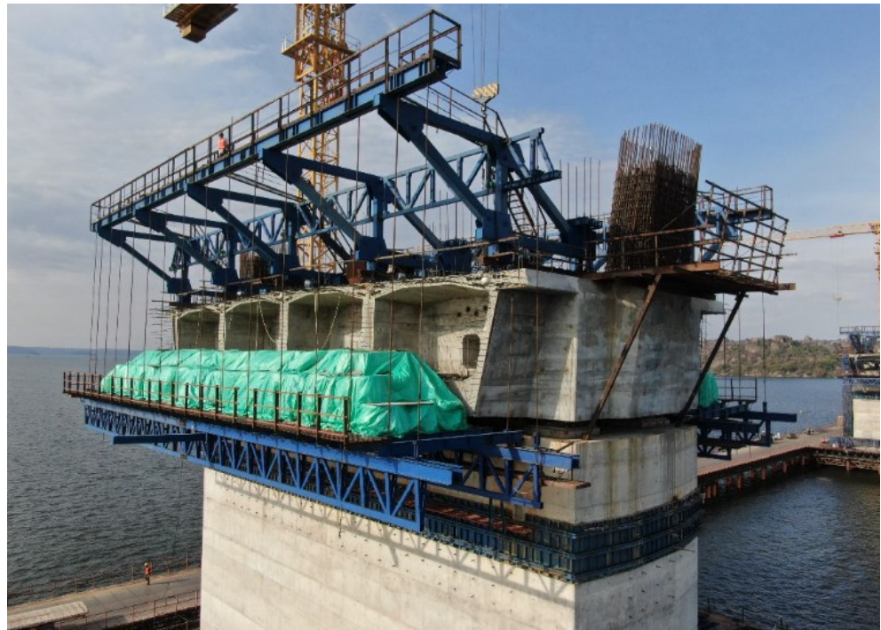
Figure 25 Testing of the form-traveller
