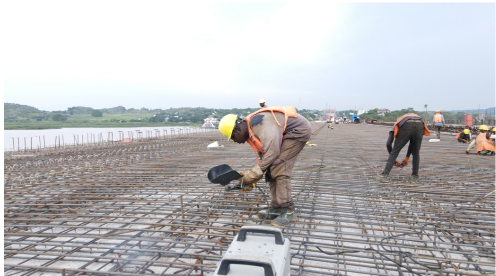
Figure 13 Reinforcement fixing prior to cast-in-place topping
