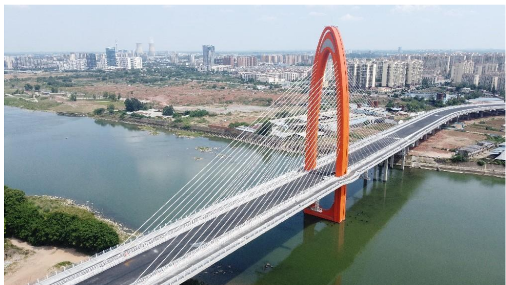
Figure 1 Huaizhou Tuojiang Bridge after being closed
