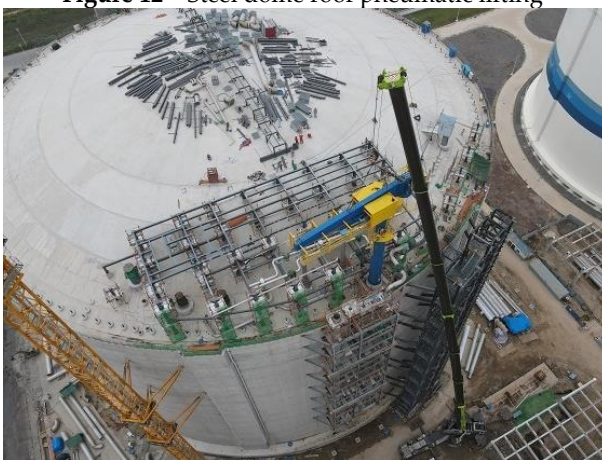
Figure 14 Installation of external equipment of tanks
