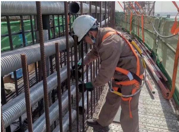
Figure 10 Tank wall construction
