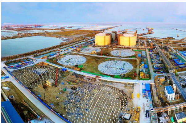
Figure 6 Pile foundation construction [12]
