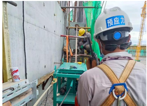
Figure 11 The lower half of the ring beam prestressed tendon tensioning
