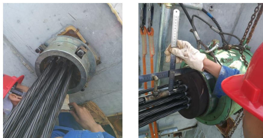
Figure 27 Friction test in the prestressed duct
