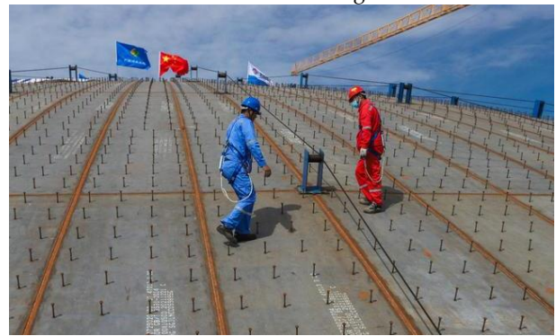
Figure 13 Concrete dome roof construction
