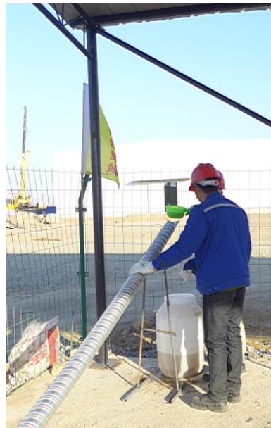
Figure 22 Pouring clear water into the ducts Figure 23 Anti-leakage performance test
