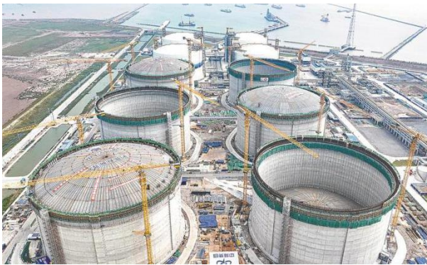
Figure 12 Steel dome roof pneumatic lifting
