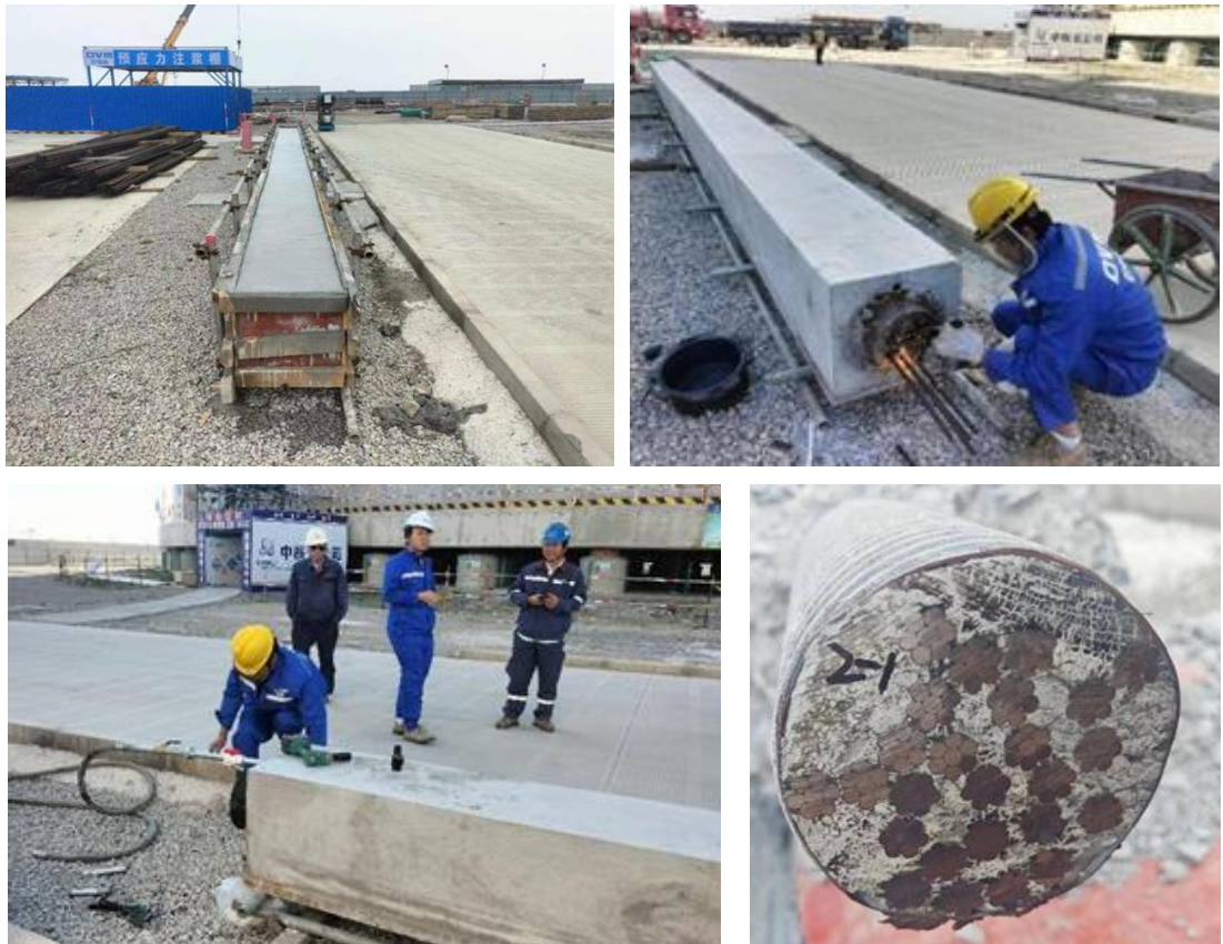
Figure 26 Full-scale grouting test in a prestressed duct
