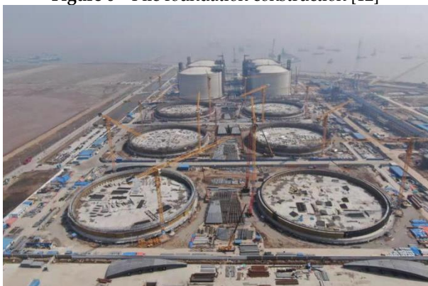
Figure 8 Tank wall construction [14]
