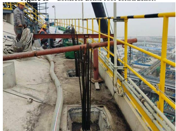
Figure 15 Tensioning of vertical prestressed tendons
