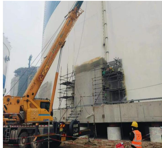
Figure 19 Prestressed tendon tensioning at the temporary opening
