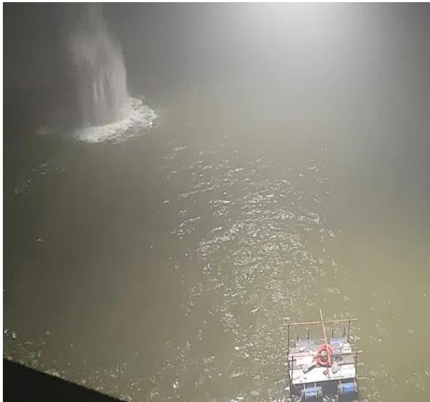
Figure 18 Water pressure test[16]
