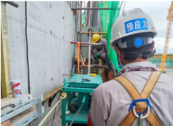
Figure 11 The lower half of the ring beam prestressed tendon tensioning
