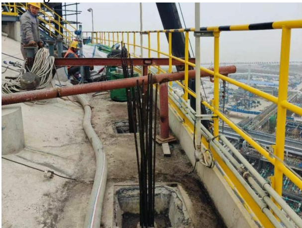
Figure 15 Tensioning of vertical prestressed tendons
