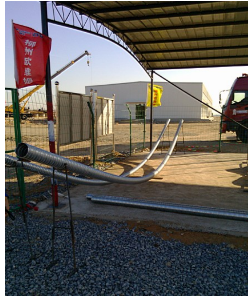
Figure 22 Pouring clear water into the ducts Figure 23 Anti-leakage performance test
