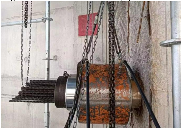
Figure 16 Tensioning of circumferential prestressed tendons
