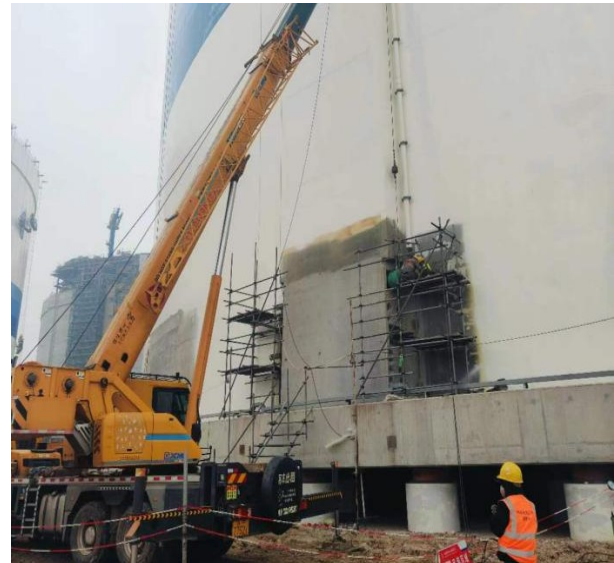
Figure 19 Prestressed tendon tensioning at the temporary opening
