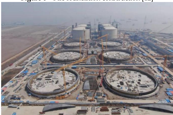
Figure 8 Tank wall construction [14]
