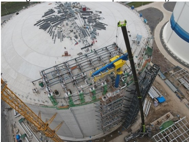
Figure 14 Installation of external equipment of tanks
