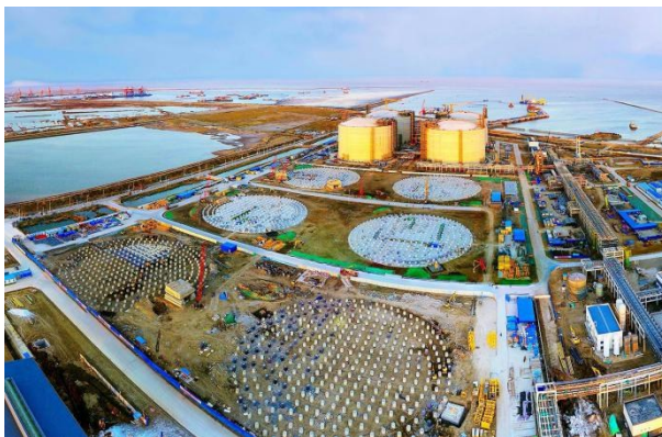
Figure 6 Pile foundation construction [12]
