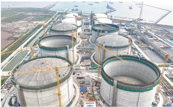
Figure 12 Steel dome roof pneumatic lifting
