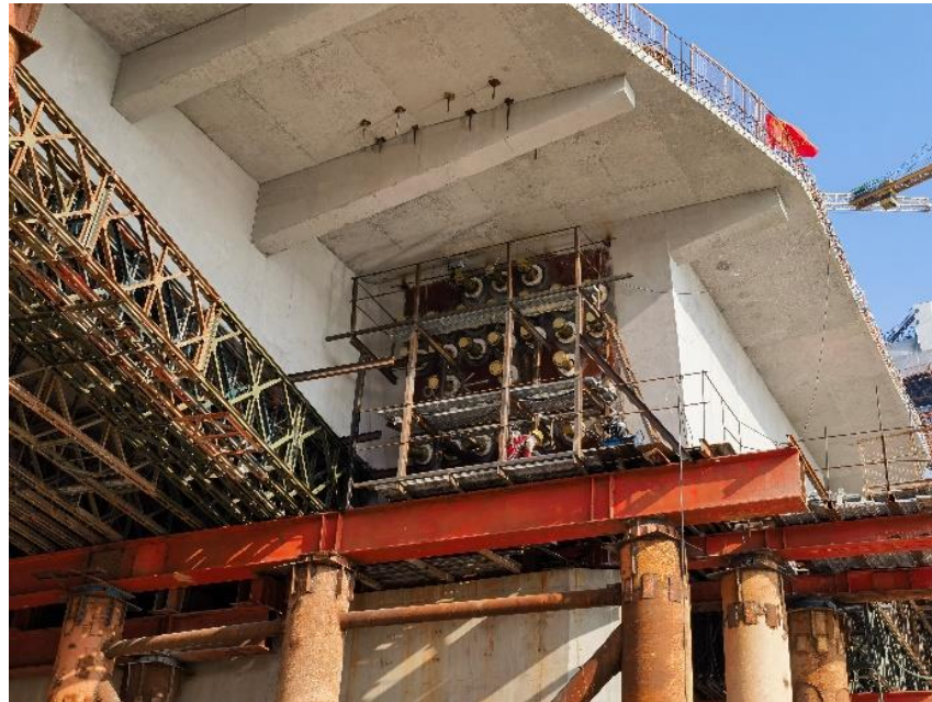
Figure 12 Photo of rear anchor surface installation
