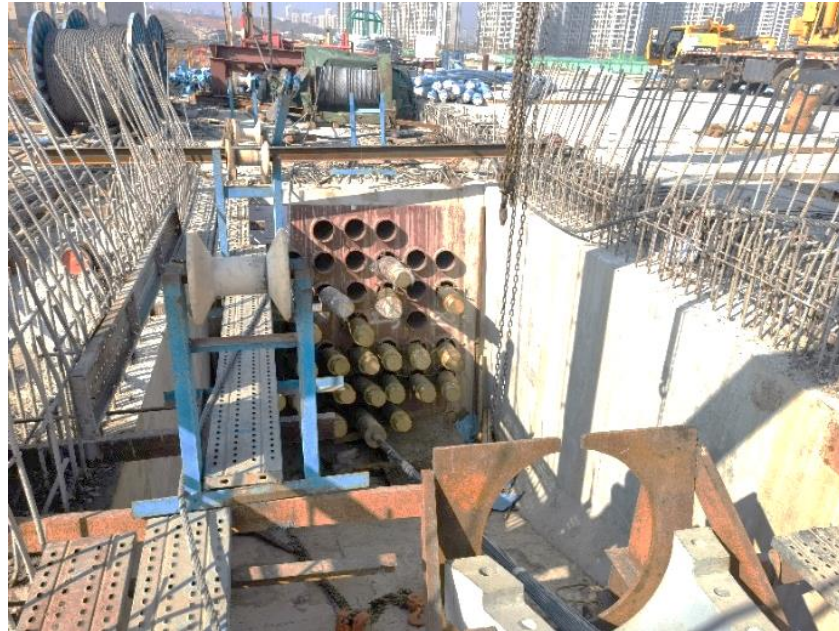
Figure 11 Installation of the first cable strand and finished cable
