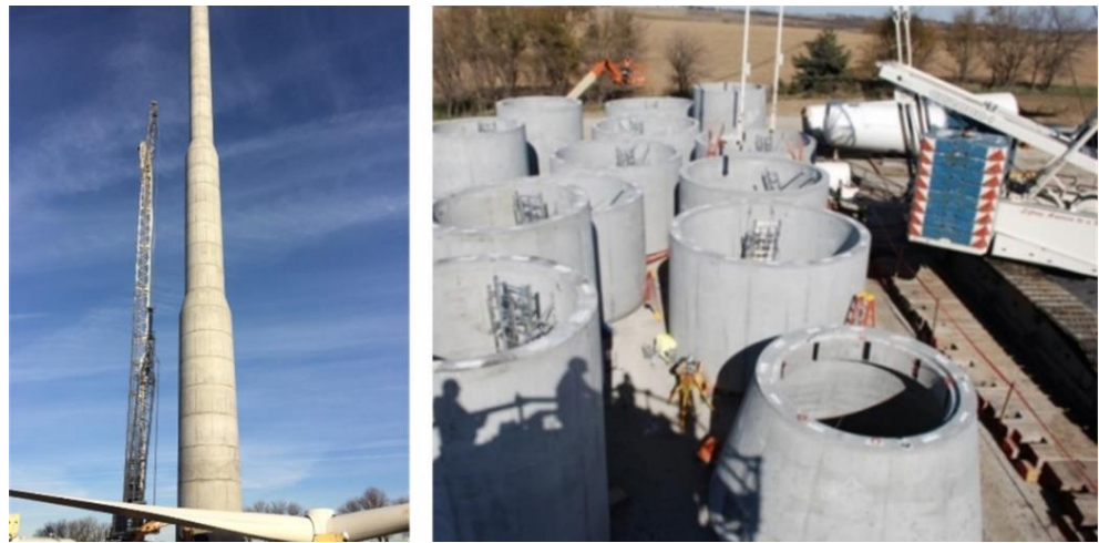
Figure 1 Full-ring precast segmental concrete wind turbine towers
