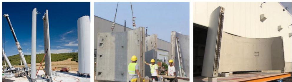
Figure 2 Precast concrete segments with vertical joints
