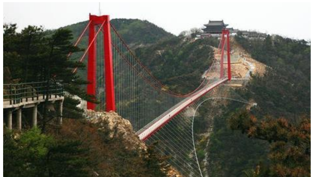
Figure 6 Yimeng Mountain pedestrian suspension bridge in Shandong Province
