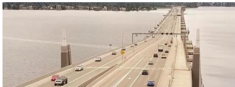
Figure 2 New SR-520 Highway Bridge, USA
