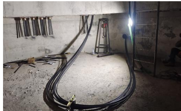
Figure 14 Strands thread in the duct from the bottom of the tower
