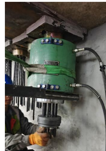
Figure 17 Tool anchor installation at the tensioning end
