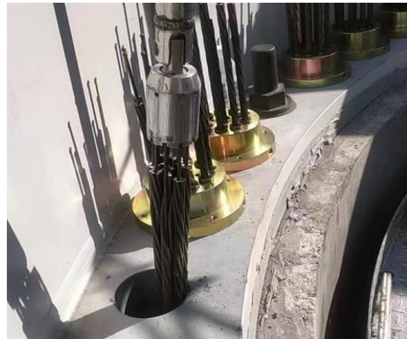
Figure 12 Strands thread out the duct from the top of the tower
