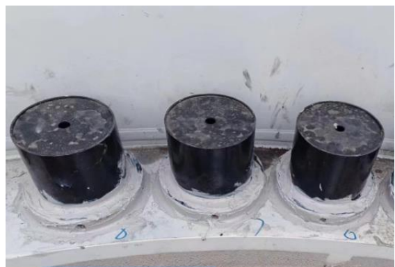
Figure 23 Installation anchorage caps
