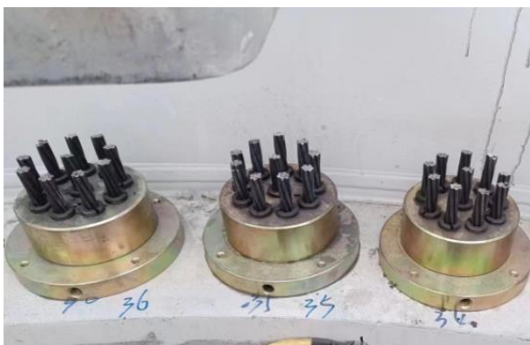
Figure 22 Cutting prestressing tensions
