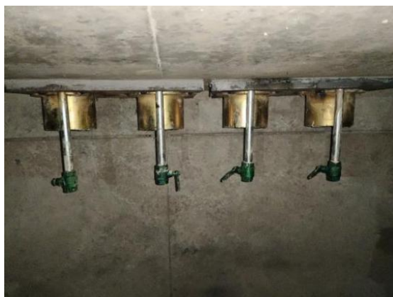
Figure 20 Installation grouting injection holes at the bottom tension end
