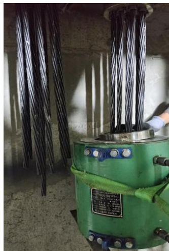
Figure 16 Jack installation at the tensioning end
