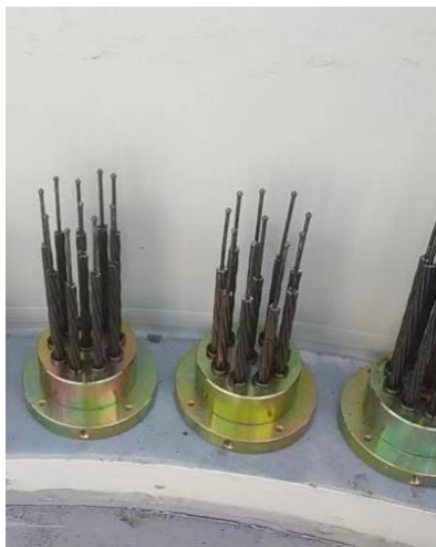
Figure 15 Dead end anchorage (Top end)
