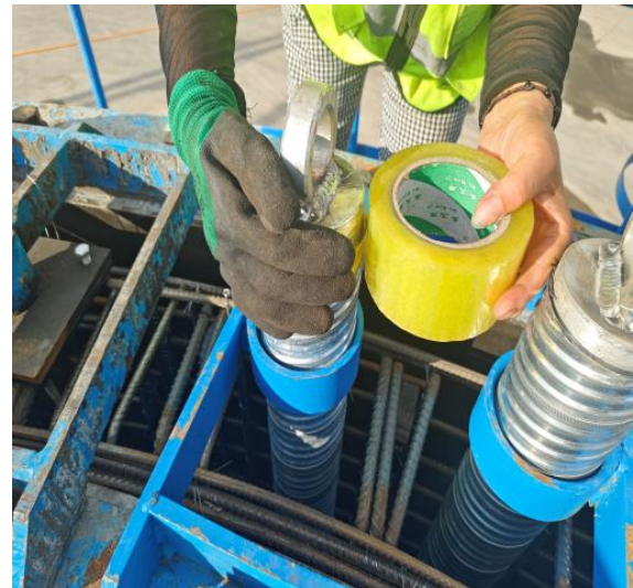
Figure 10 Sealing the top of the metal corrugated duct
