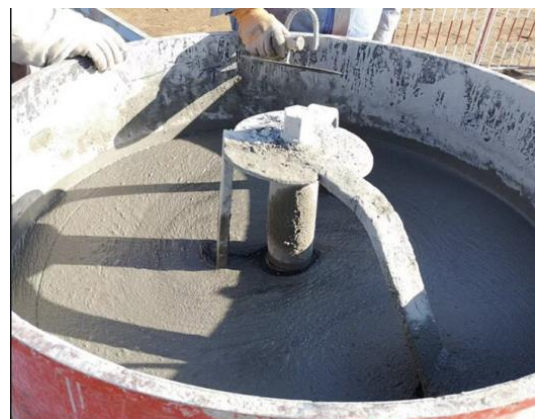
Figure 21 Mixing grouting material
