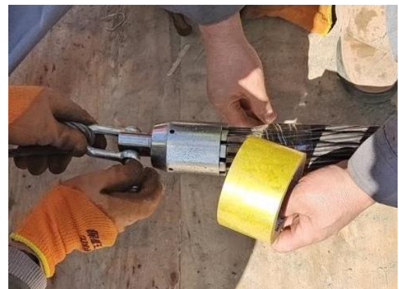
Figure 8 Wrapping steel strand at pulling head
