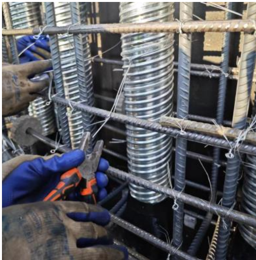
Figure 9 Fixing the bottom of the metal corrugated duct
