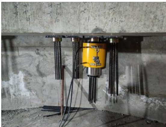
Figure 18 Tensioning prestressing tendons
