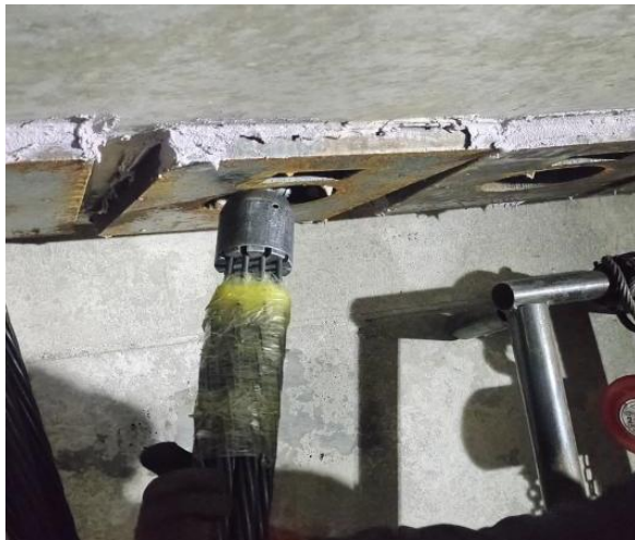
Figure 11 Strands thread in the duct from the bottom of the tower
