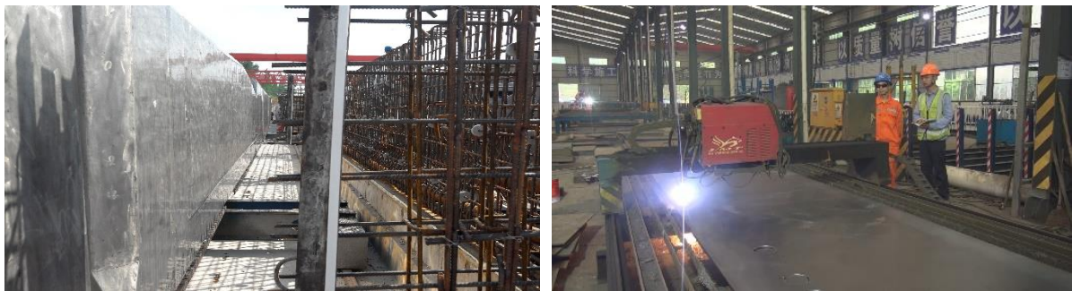
a) Composite stainless-steel plates b) Plasma cutting of embedded steel plates
