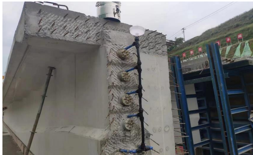
Figure 11 Arrangement of continuous grouting
