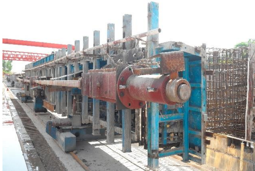
Figure 8 Automatic sliding hydraulic integral formwork
