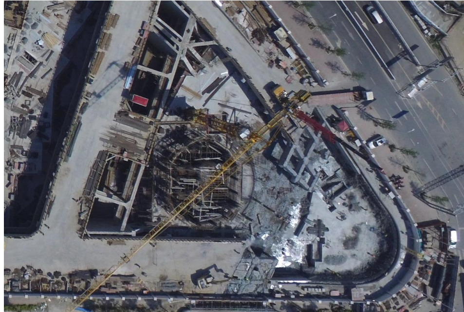
Figure 8 Actual picture of early backfill construction
