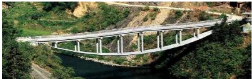
Figure 7 Dongkou Bridge in Shaoyang, Hunan Province
