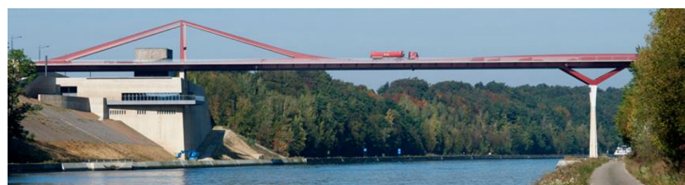
Figure 5 Fronhoven Bridge (cable-stayed - umbrella truss collaboration), Belgium
