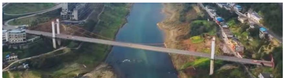
(a) Wujiang Bridge of the Zhanan line in Guizhou (stayed cable-suspension collaboration)
