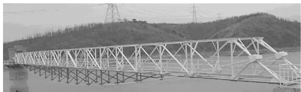
Figure 9 Pedestrian bridge at Muchengtang Reservoir
