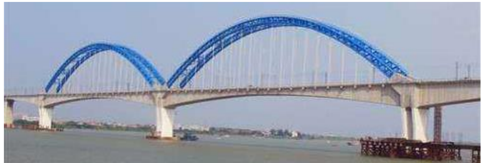
(b) Xijiang Bridge of the Guangzhou-Zhuhai Railway (arch-rigid frame (beam) collaboration)
