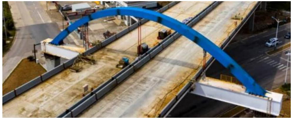
Figure 6 Zhoudaiyadong Bridge (arch-beam collaboration), China
