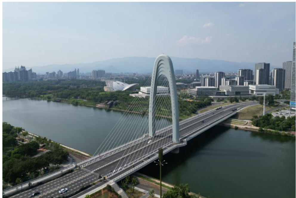
Figure 3 Image of the Jinwu Bridge after it was completed
