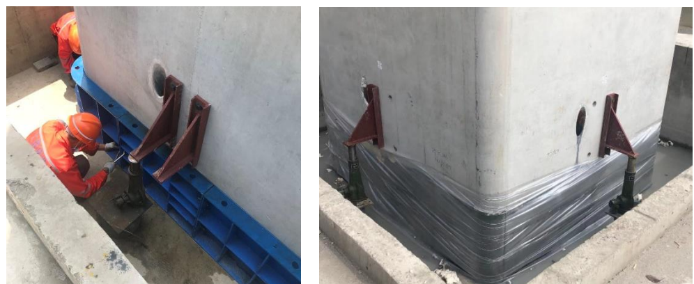
(a) Formwork installation
