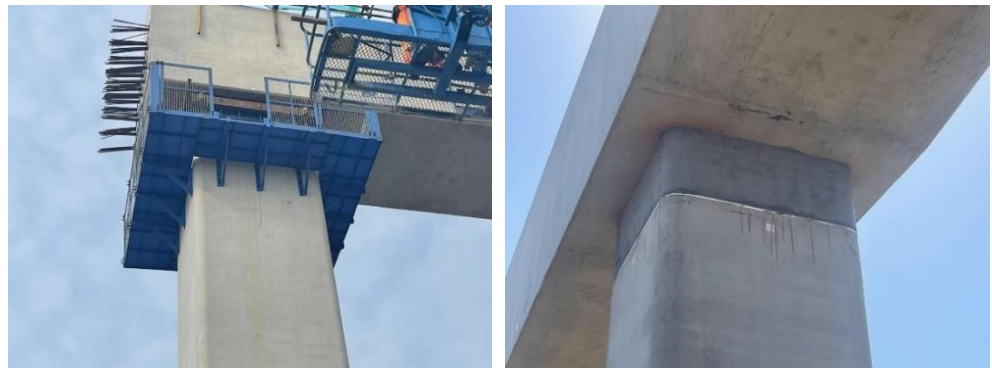
(a) Formwork and guardrail installation (b) Formwork dismantling and maintenance
