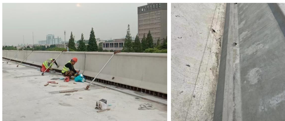
(a) Before forming the wet joint (b) After forming the wet joint
