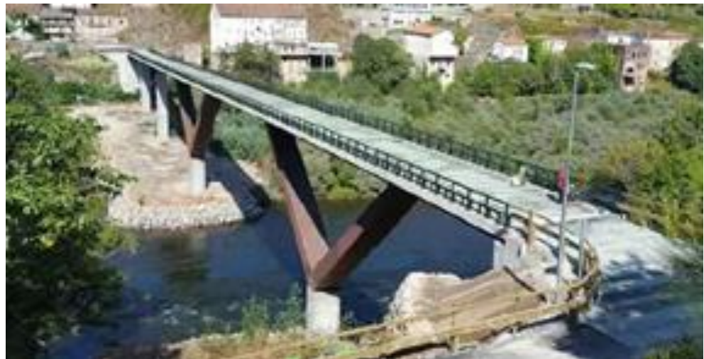
Figure 8 Minho River Bridge, Spain
