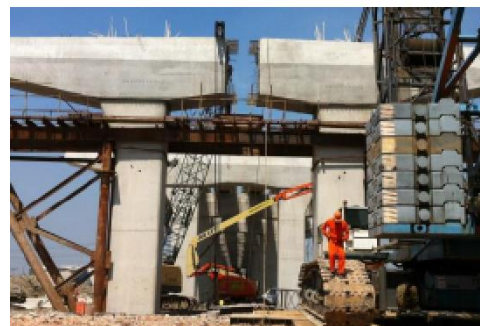
(a) Post-pouring belt bent cap
