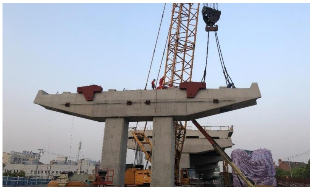
Figure 11 Construction of the Shanghai S26-5 bent cap hanging lock method
