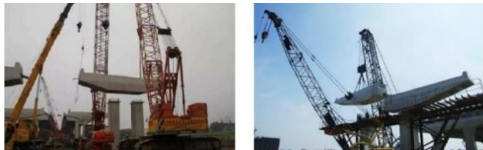
(a) Whole prefabricated bent cap
