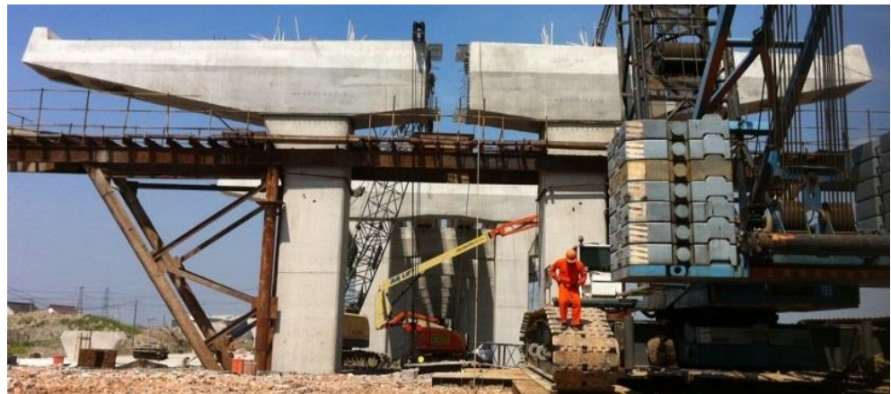
Figure 8 S26 Two-section precast bent cap construction
