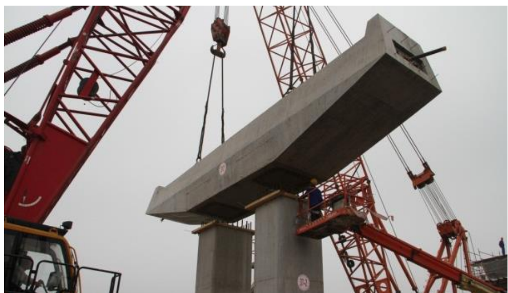
Figure 7 Construction of the bent cap of the Shanghai S6 highway project
