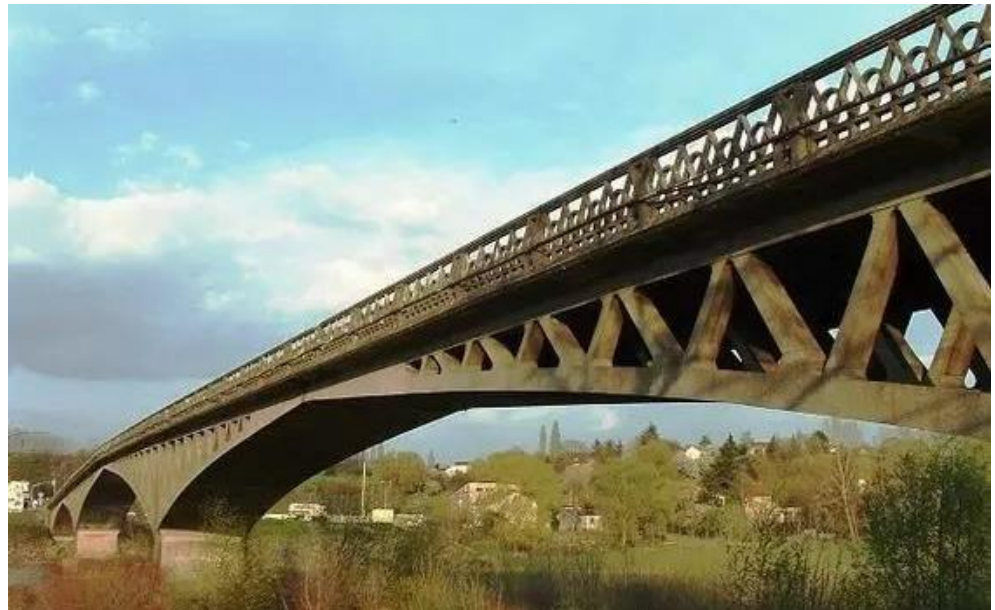
Figure 4. The Veudre Bridge
