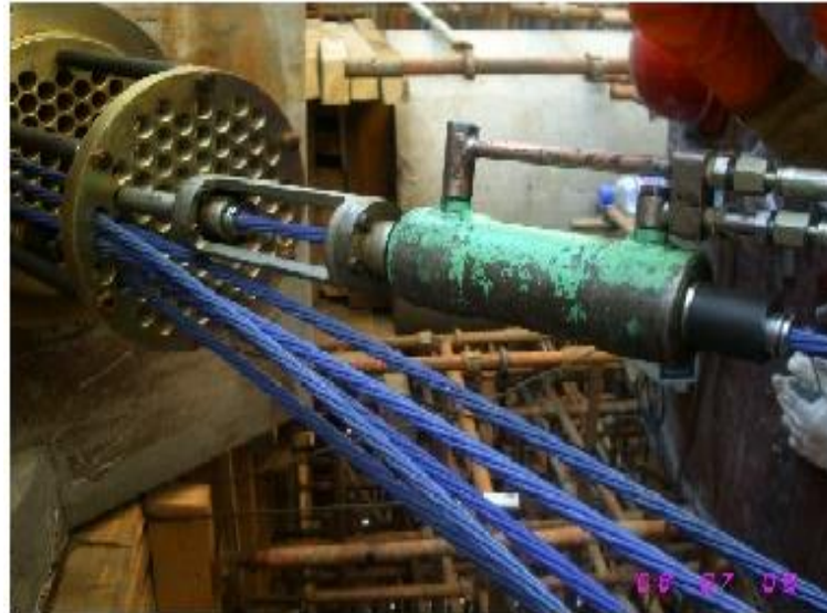
Figure 5. On-site tensioning of a single strand
