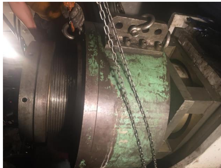
Figure 6. On-site overall tensioning of cables
