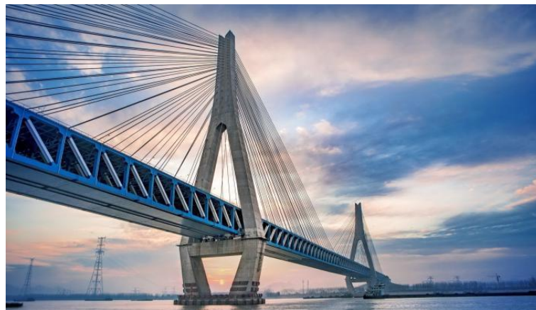
Figure 1. Tongling Rail-cum-Road Changjiang River Bridge
