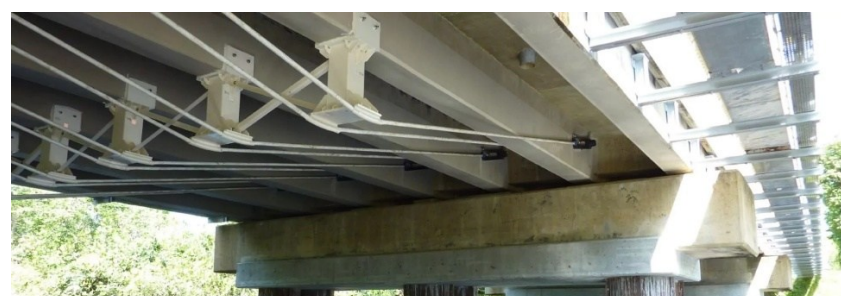
c) application in bridges
