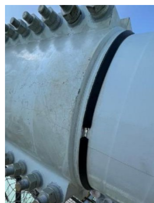
Figure 17 Sealing sample of the cable clamp ring seam
