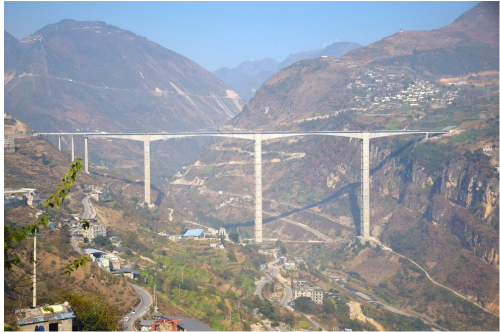
Figure 1 Jinyang River Bridge in Jinyang County
