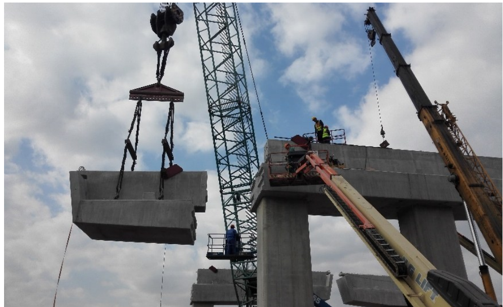
Figure 10 Construction of a three-section bracket joint bent cap of S7 in Shanghai
