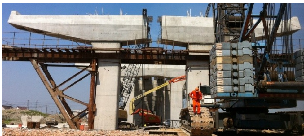
Figure 8 S26 Two-section precast bent cap construction
