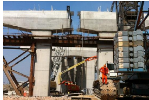
(a) Post-pouring belt bent cap
