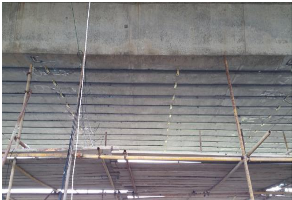
Figure 2 Bridge bottom after reinforcement
