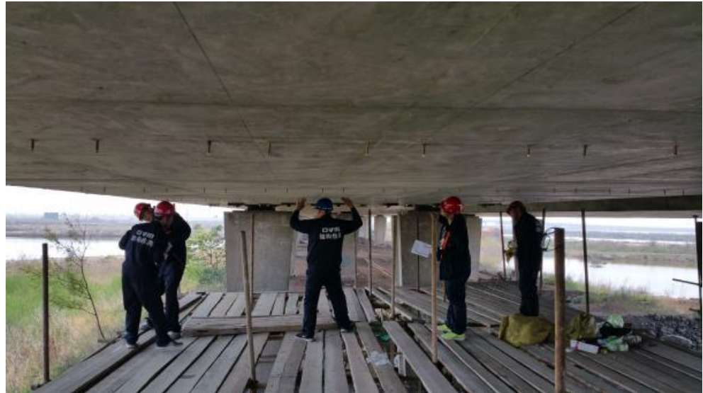
Figure 1 Bridge bottom before reinforcement
