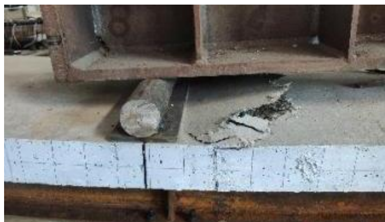
Figure 8. Concrete slab failure form of the third beam
